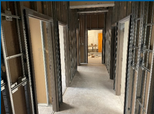
New office/conference room door frames and walls installed
